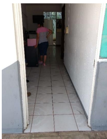
Puerta exterior – D.I.F. Municipal
