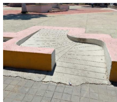
Rampas – Plaza Principal
